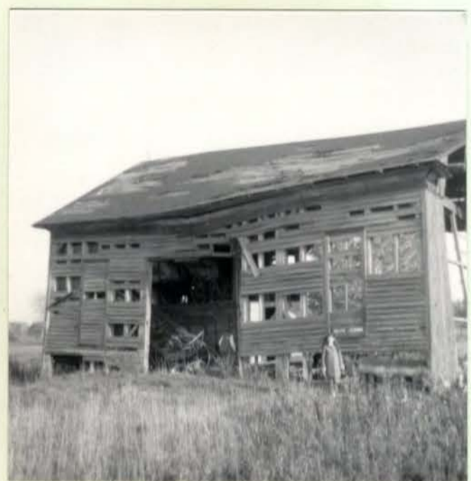
This is the original church which Daniel Patterson bought and used as a barn. It was torn down and the remains burned around 1980.
